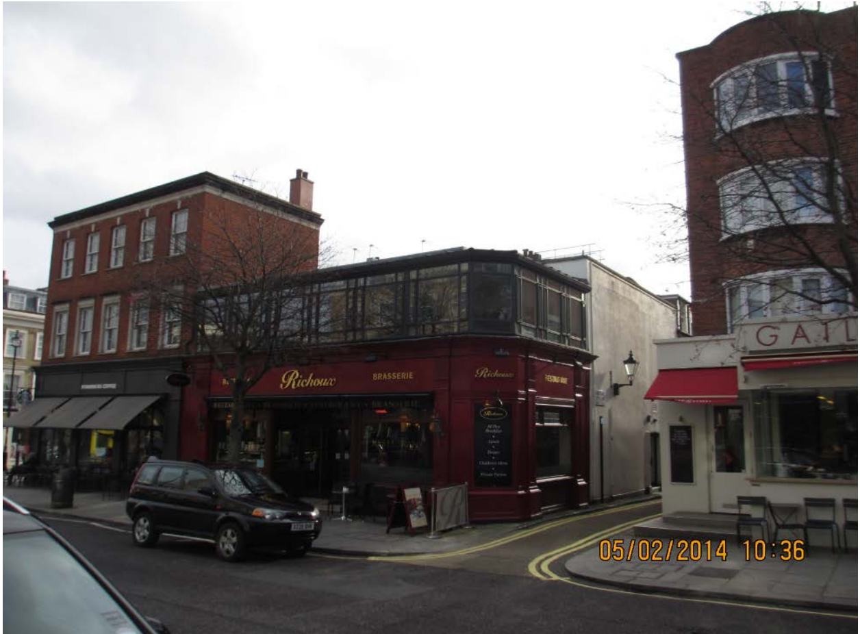
Application site as seen from Circus Road.
